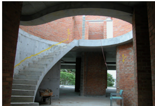
The feature stair has taken shape.
