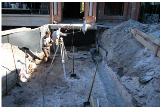
Preparation for driveway slab and adjacent reinforced concrete block retaining wall.
