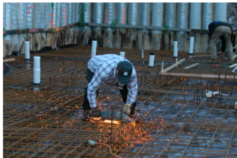
The final touches. Concrete cover (thickness) to reinforcement is important.
