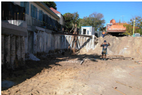
Excavation for the lower ground floor is complete.
