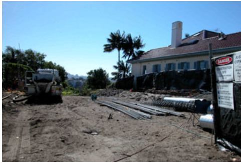
The site is cleared and prepared for the start of construction.
