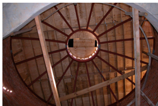
The steel framed dome in place.
