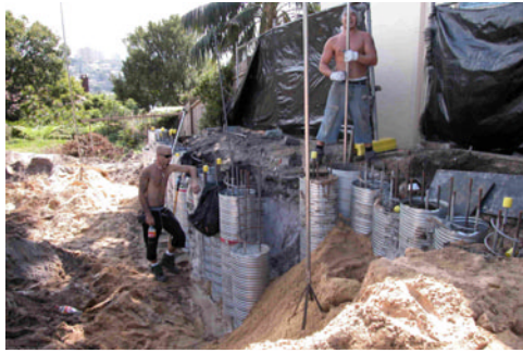
The process of concrete piling is carried out.
