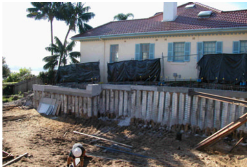
The concrete pile retaining wall is finished complete.
