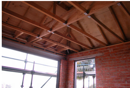
The conventionally framed timber roof structure.
