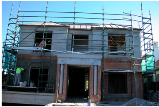
Finishes being applied.
